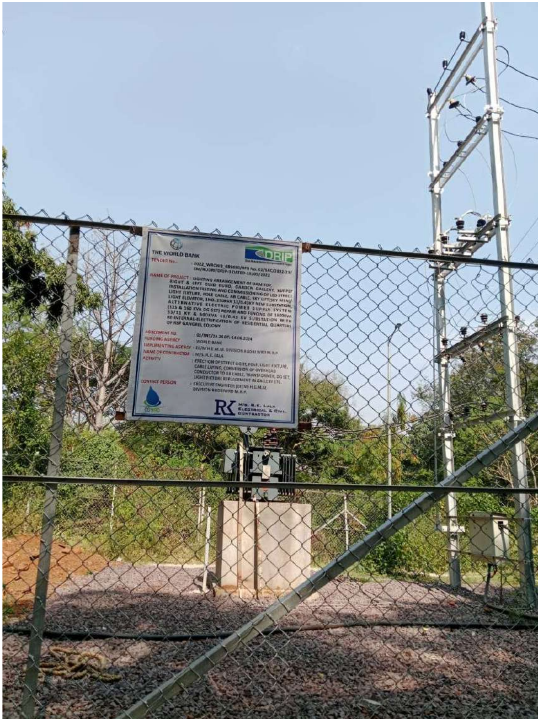
Display Board at Site
